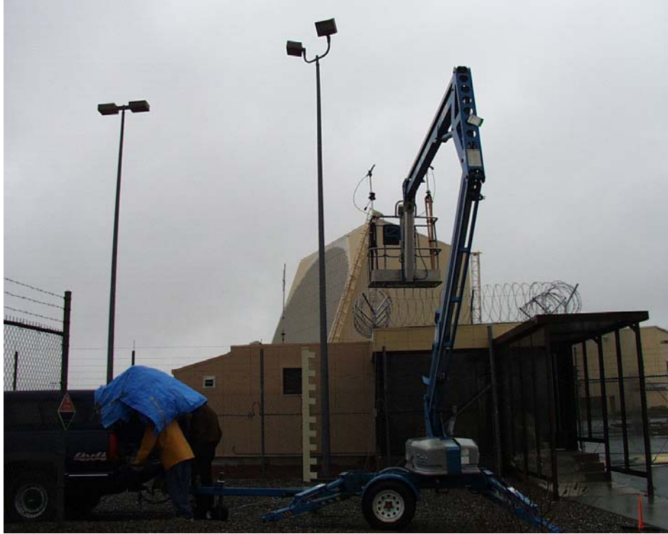
Photograph 3: Test Point 12 – Entry Control Point
